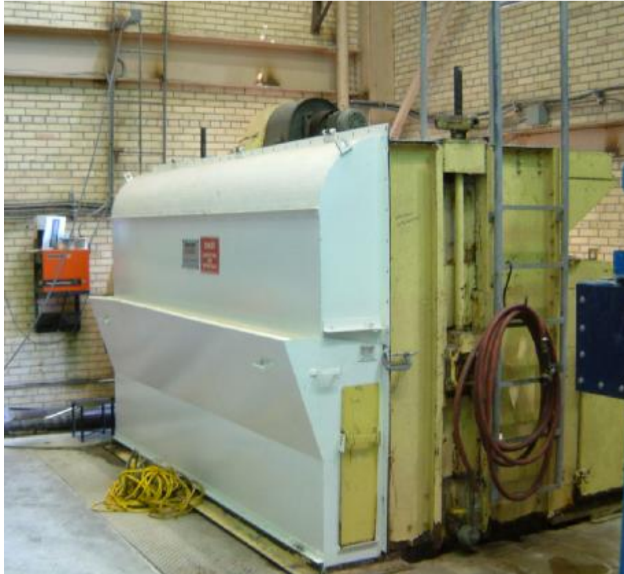
Figure 4-4 QE Low Lift Traveling Screen
