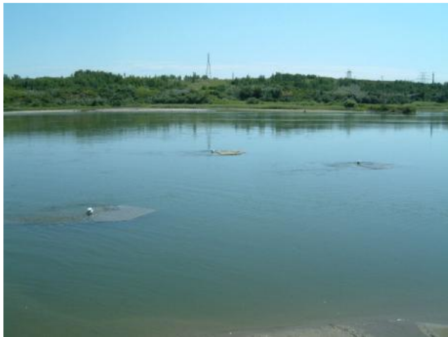
Figure 4-2 QE Low Lift Intake Structures
